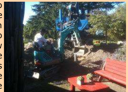
Drilling new soak holes!
