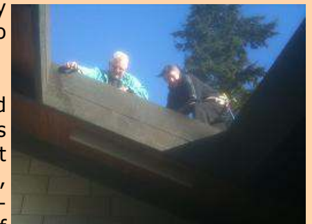
Carpenters Steve and Dean work on the camp kitchen skylight
